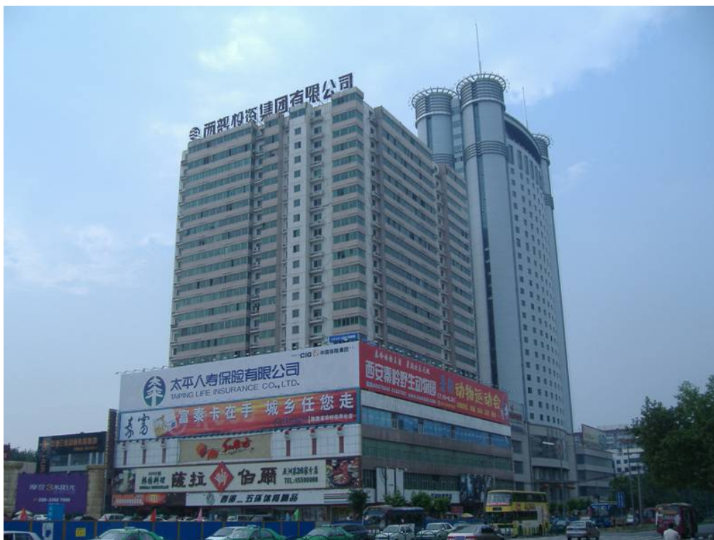
Outside Wall: South
